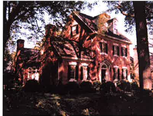
Beautiful, established houses are typical of the Twickenham area.
